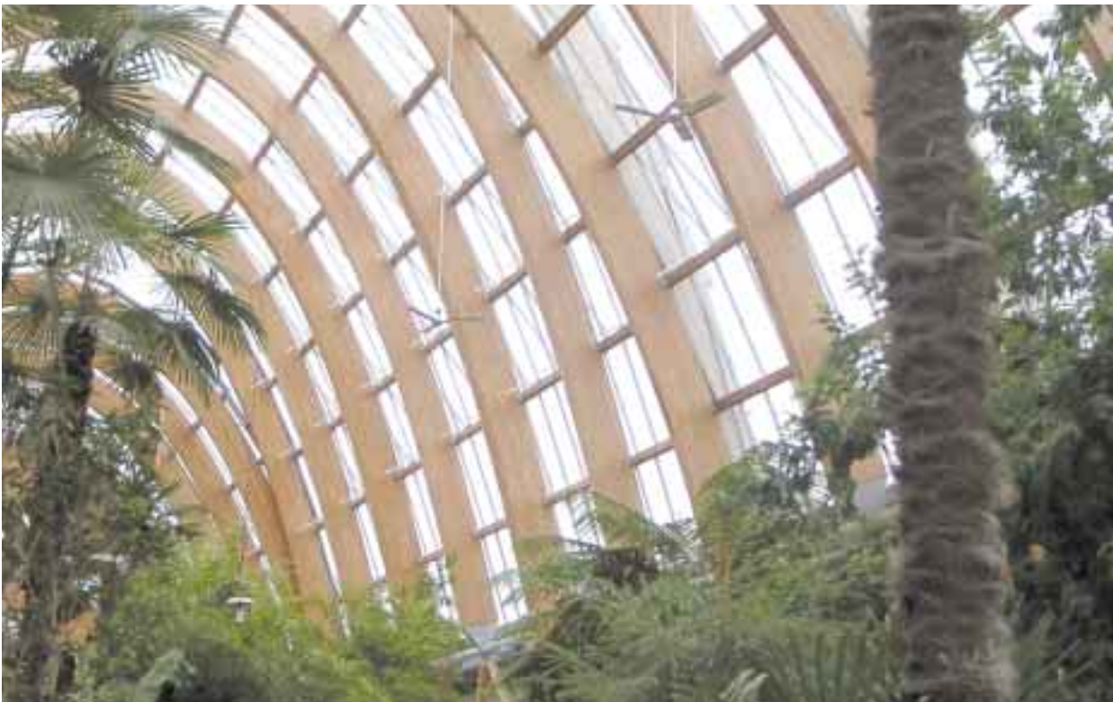
The Winter Gardens, Sheffield. The use of timber in construction is increasing and can make a dramatic visual impact.
