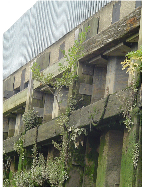
Plant communities colonising the wall ledges and timber fenders at Deptford Creek (photo © Simon Hoggart and Robert Francis, KCL).
