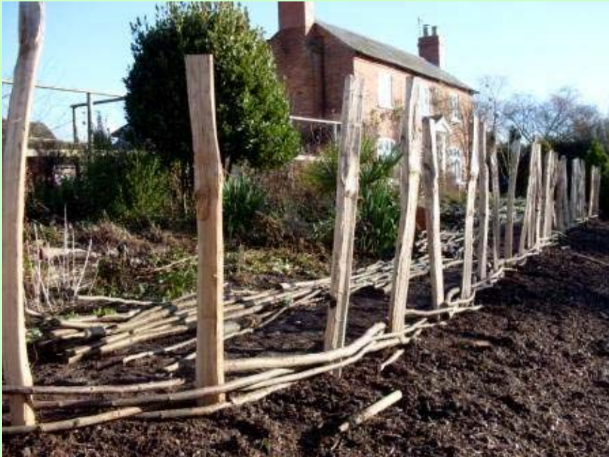
Continuous weave fencing by a SWOG member
