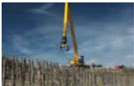
The installation of sweet chestnut fixing posts up to 4m long. These were installed into sloping mud banks using a long-reach excavator.
