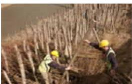
The cross-hatching of long hazel faggots between the posts to create cavities for the trapping of sediment. 6,000 faggots were used in this project to fill a cavity 200m x 4m x 25m.
