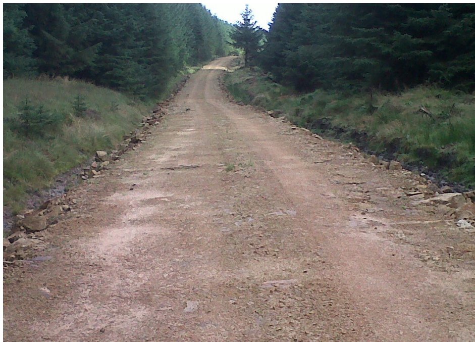
An example of the roads that will - thanks to their new grant - be laid down at Whitelyne
