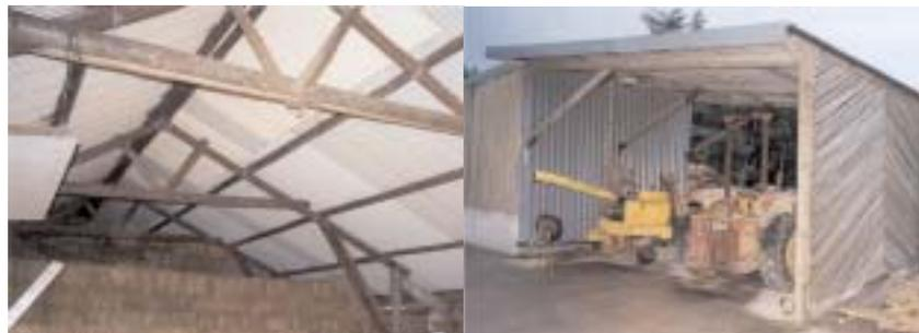
The use of round timber is increasing in semi-rural commercial buildings and visitor centres. Commonly, round elements are used as columns and bracing as well as roof members. Sawn timbers may then be used as principal beams, floor joists and for cladding.
