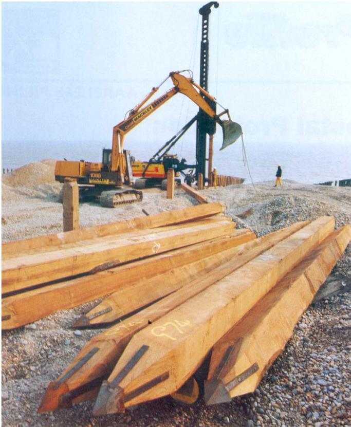
**Figure 3: Timber piles being installed for beach protection
