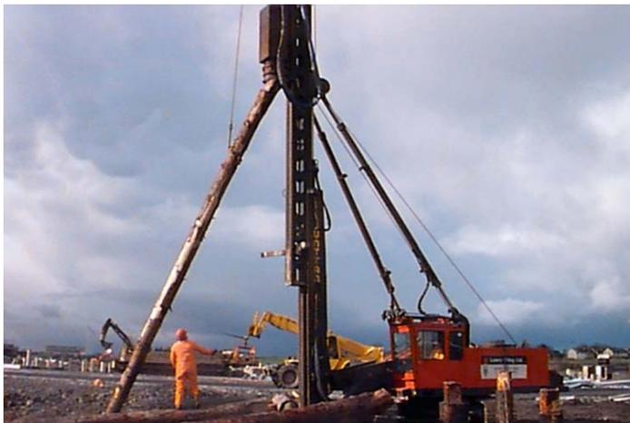
**Figures 4 and 5: Irish grown Sitka spruce logs being used for pilings (photos courtesy of P.Quigley/NUI)**
