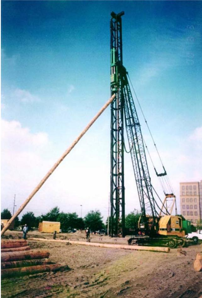
**Figure 10: Pile installation (photo courtesy Kardon piling)**
