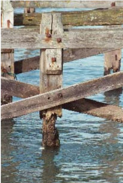
**Figure 6: Marine borer attack on 120 year old greenheart pile**
