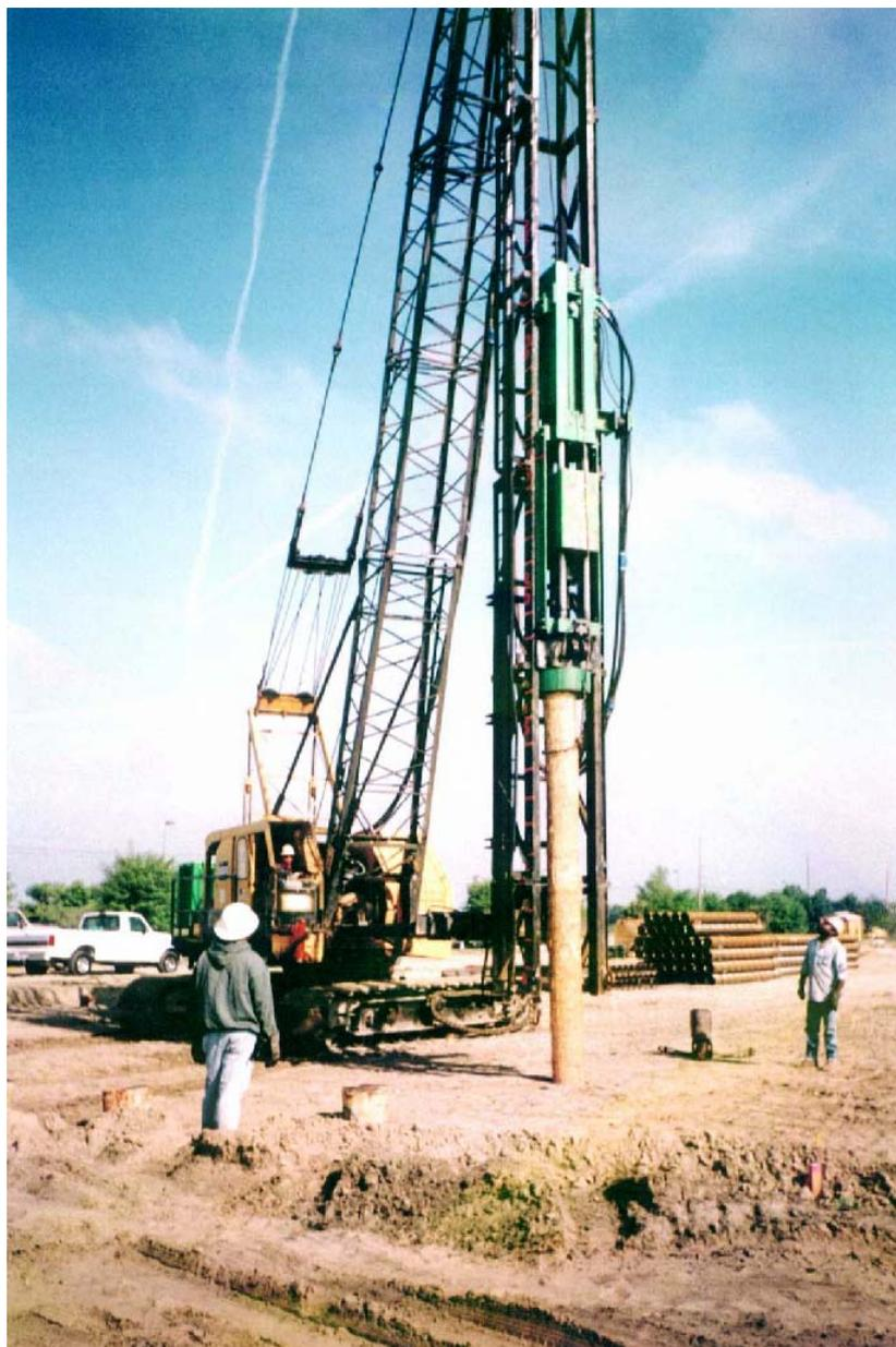
**Figure 9: Timber pile driving** (photo courtesy Kardon Piling)
