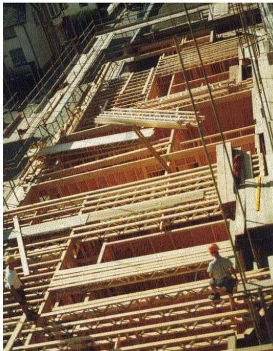
**Floor construction using metal web timber beams**
