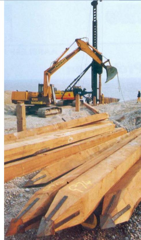
Although timber piles are rarely used on shore in the UK, in other countries notably the United States, Canada and Australia, they are used widely. For many structures, timber piles are a highly suitable choice of foundation, given appropriate ground conditions. They are economical, easy to transport, handle, cut to length and work with on site; and particularly suited for locations with access difficulties, or where excavations and the delivery of concrete would pose problems.
