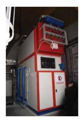
In the case of larger boilers, the fuel quality is determined by the boiler requirements. Wood chips with a water content of less than 30% can often present a problem
