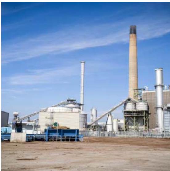
Semcorp biomass plant in Middlesbrough
