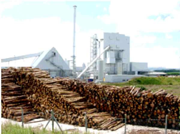
The E.ON plant at Lockerbie
