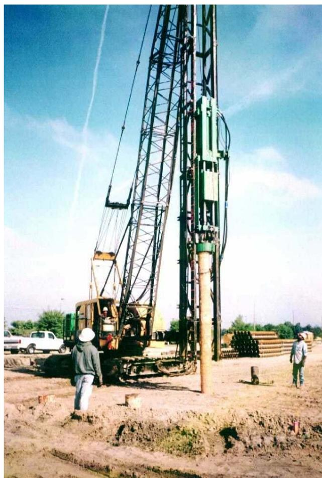
**Figure 5** Timber pile driving (Photograph courtesy of Kardon Piling)
