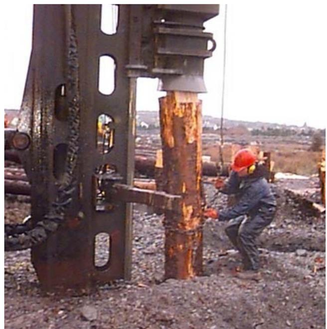
**Figure 3** Irish grown Sitka spruce logs being used for pilings (Photographs courtesy of P.Quigley/NUJ)
