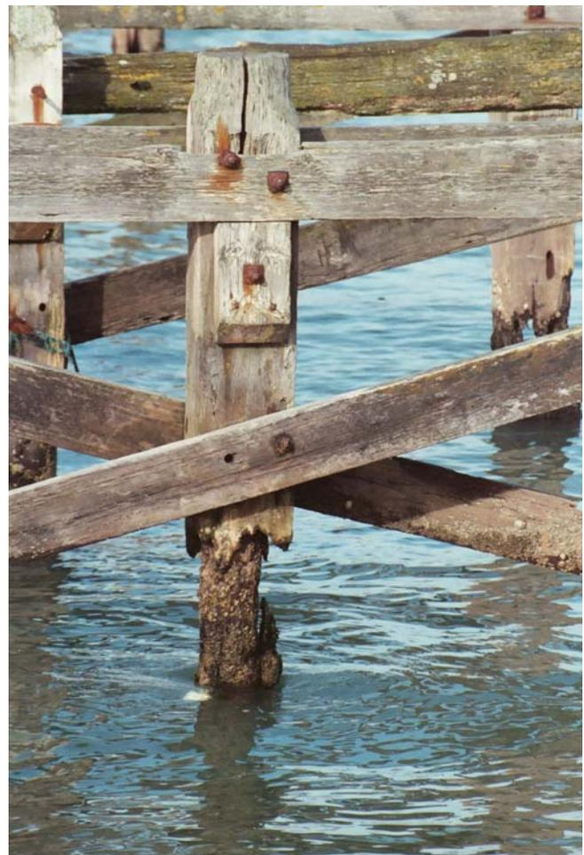
**Figure 4** Marine borer attack of an 120 year old greenheart pile
