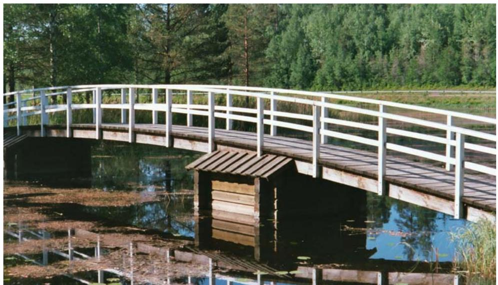
**Figure 9** Footbridge at Garpenburg, Sweden, with timber foundation piers
