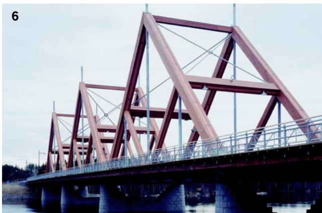
Figures 5 and 6 Vihantasalmi Bridge, Finland. Glue laminated timber trusses, each spanning 42 m (Photos courtesy of the Nordic Timber Council)
