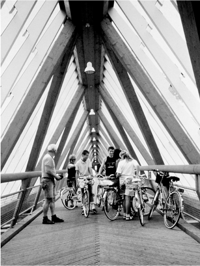
Figure 4 Bridge across the River Neckar, Remseck, Germany (Photo courtesy of the Nordic Timber Council)
