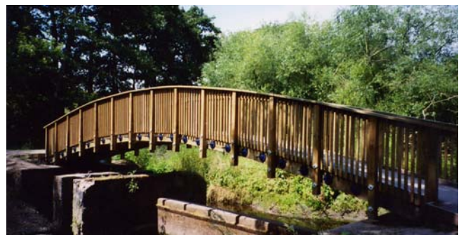
Figure 10 Timber arch bridge near Northwich, Cheshire
