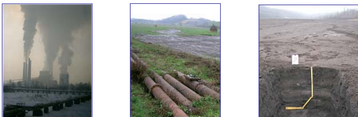
Figure 1. The thermo-electric power plant in Tuzla, pipelines for wet deposition of coal ash and an ash profile on a recently abandoned coal ash deposit.
