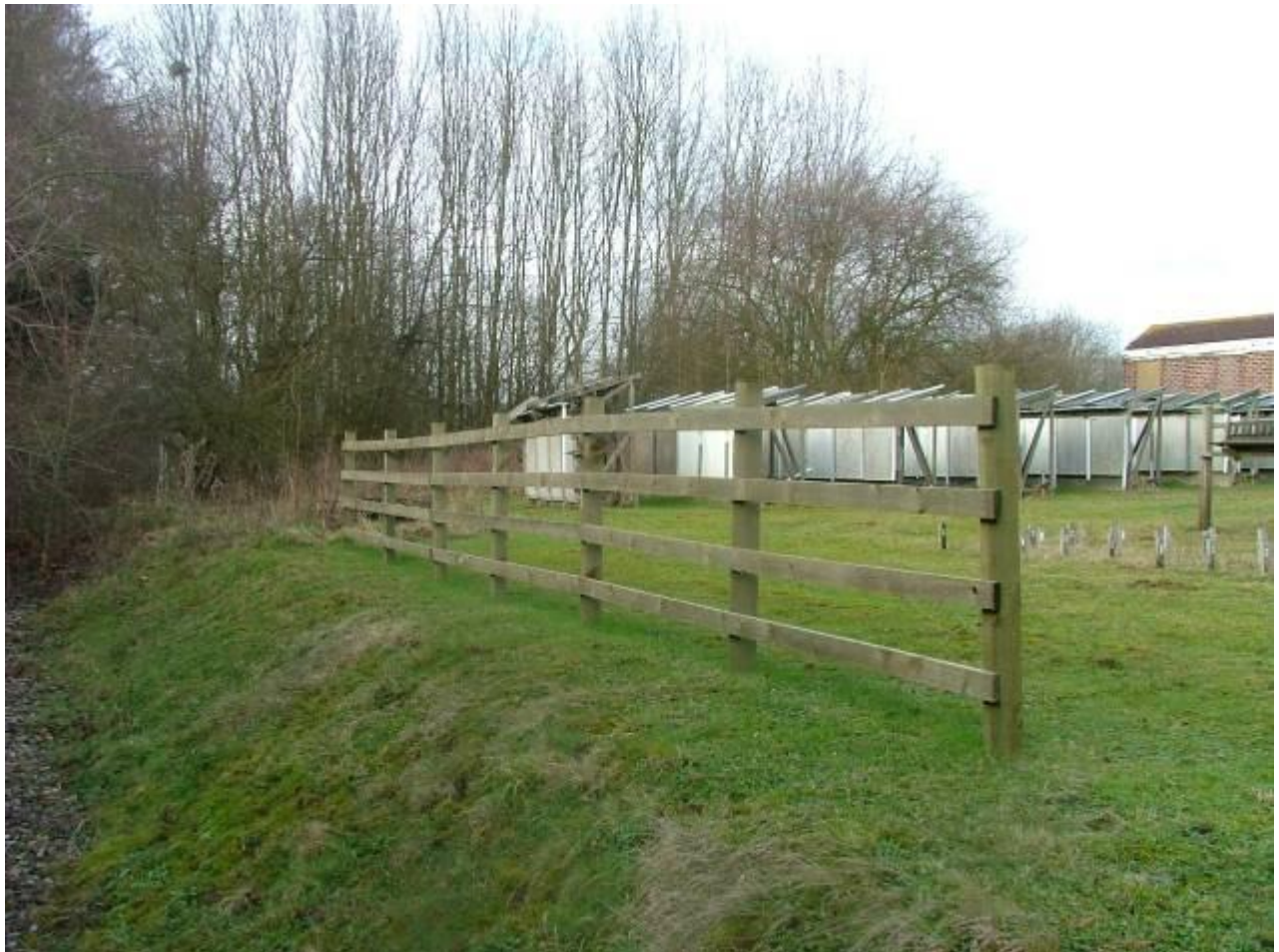
Figure 4: Incised timber fencing erected at BRE, Garston.
