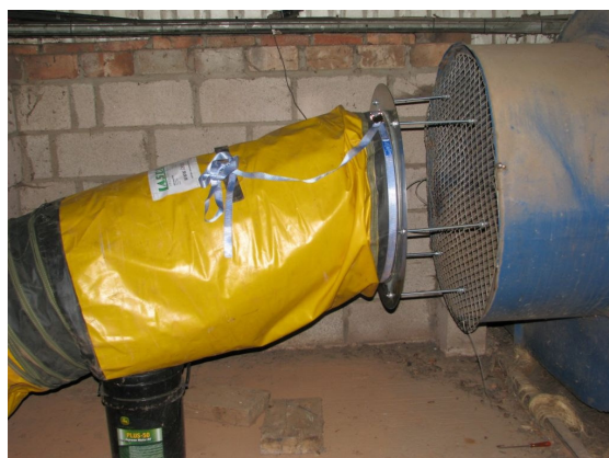
Drying fan connected to hot air pipe
