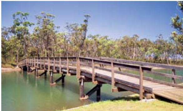
Figure 5: Footbridge on timber pilings (photo courtesy of Outdoor Structures Australia)
