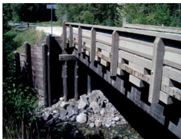
Figure 1: Road bridge supported on timber piles and abutments near Whistler, British Columbia, Canada (photo courtesy of G Freedman)
