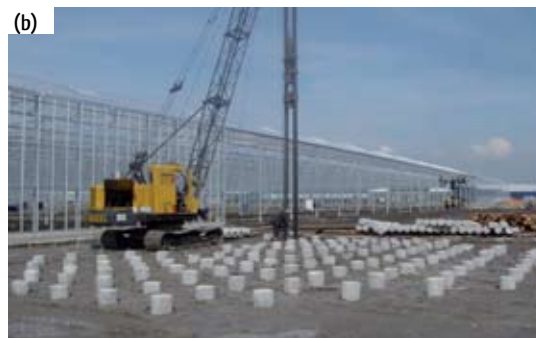
Figure 4: (a) and (b) Timber piling with concrete extensions (photos courtesy of Willem van Delft/D van Biezen B.V.)
