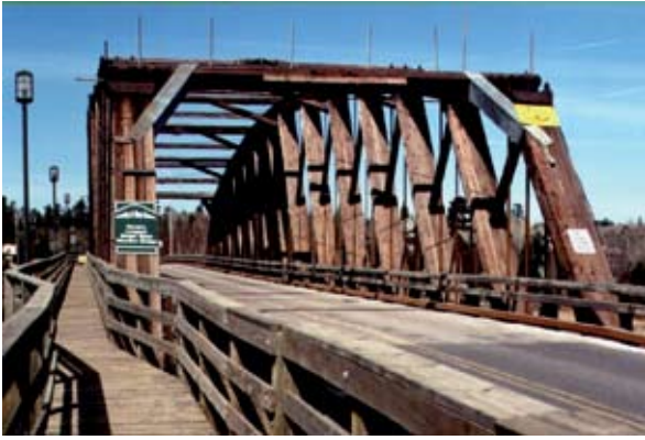
Figure 2: Sioux Narrows Bridge, Ontario, Canada built in 1936 from incised, creosoted Douglas fir. Still in use as a single lane highway bridge (photo courtesy of Ben J. Haight)
