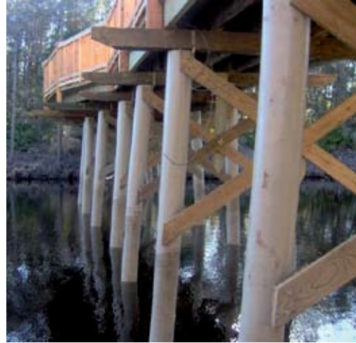
Figure 7: Polymer coated timber piling (photo courtesy of CMI)
