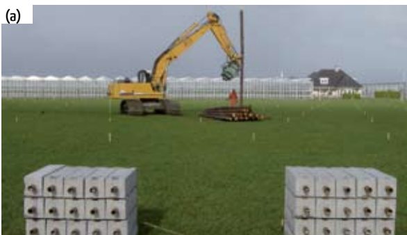
Figure 4: (a) and (b) Timber piling with concrete extensions (photos courtesy of Willem van Delft/D van Biezen B.V.)
