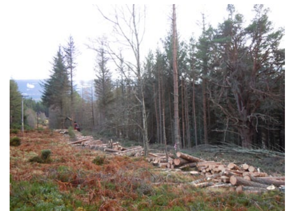
Harvester widening the powerline wayleave.
