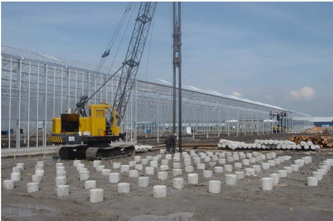
**Figure A1: Timber piles with concrete extensions being installed for a water tank in Holland (photo courtesy of D. van Biezen B.V.)**
