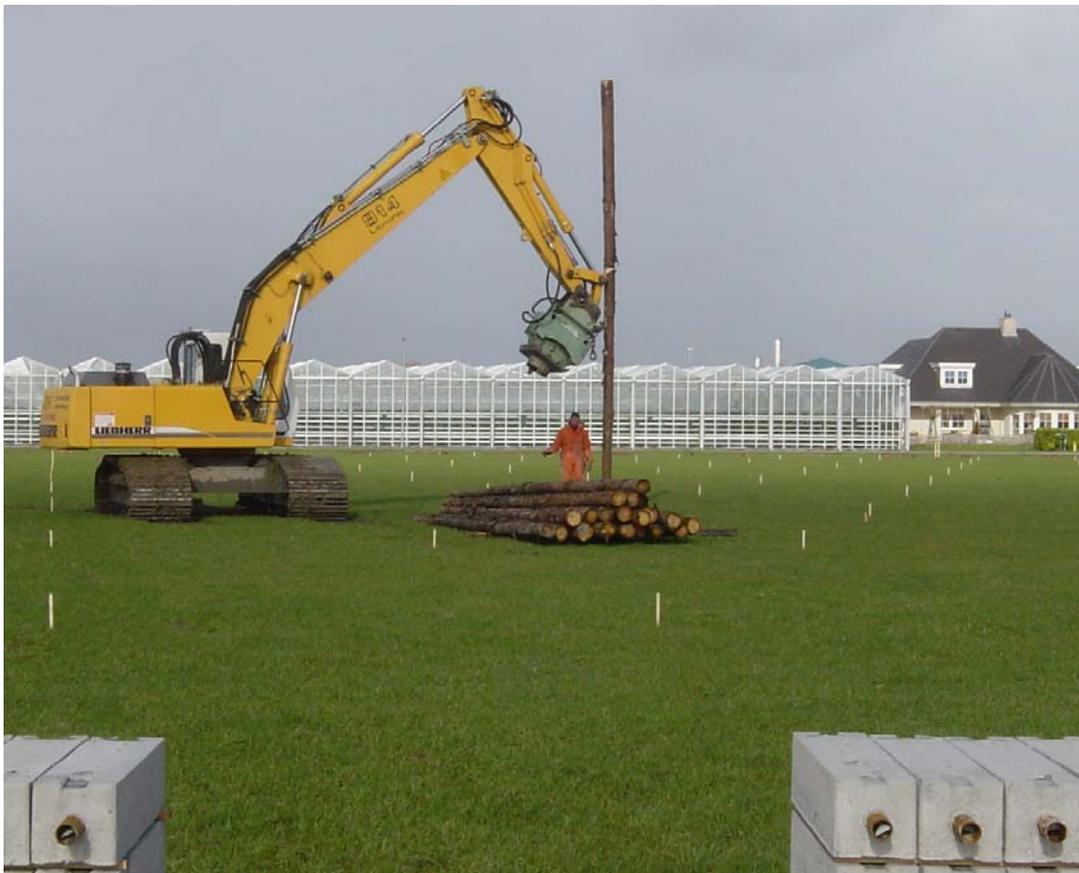
**Figure A2: Timber piles being driven into soft ground using the arm of an excavator, with square section concrete extensions in foreground. (photo courtesy of D. van Biezen B.V.)**
