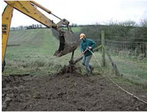
Removing soil from excavated root system using compressed air
