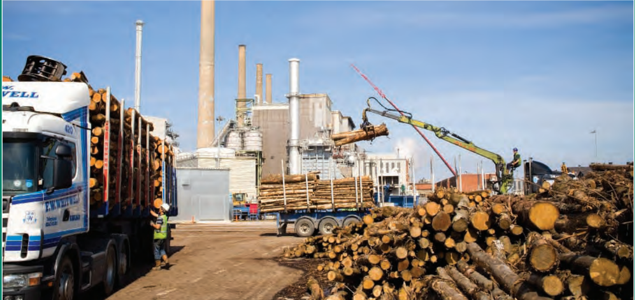
The Wilton 10 Biomass Power Station
