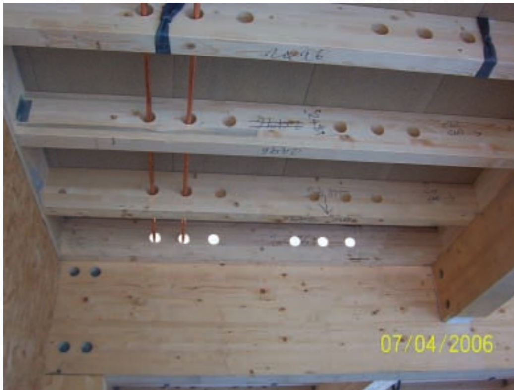
Gluelaminated timber structure
