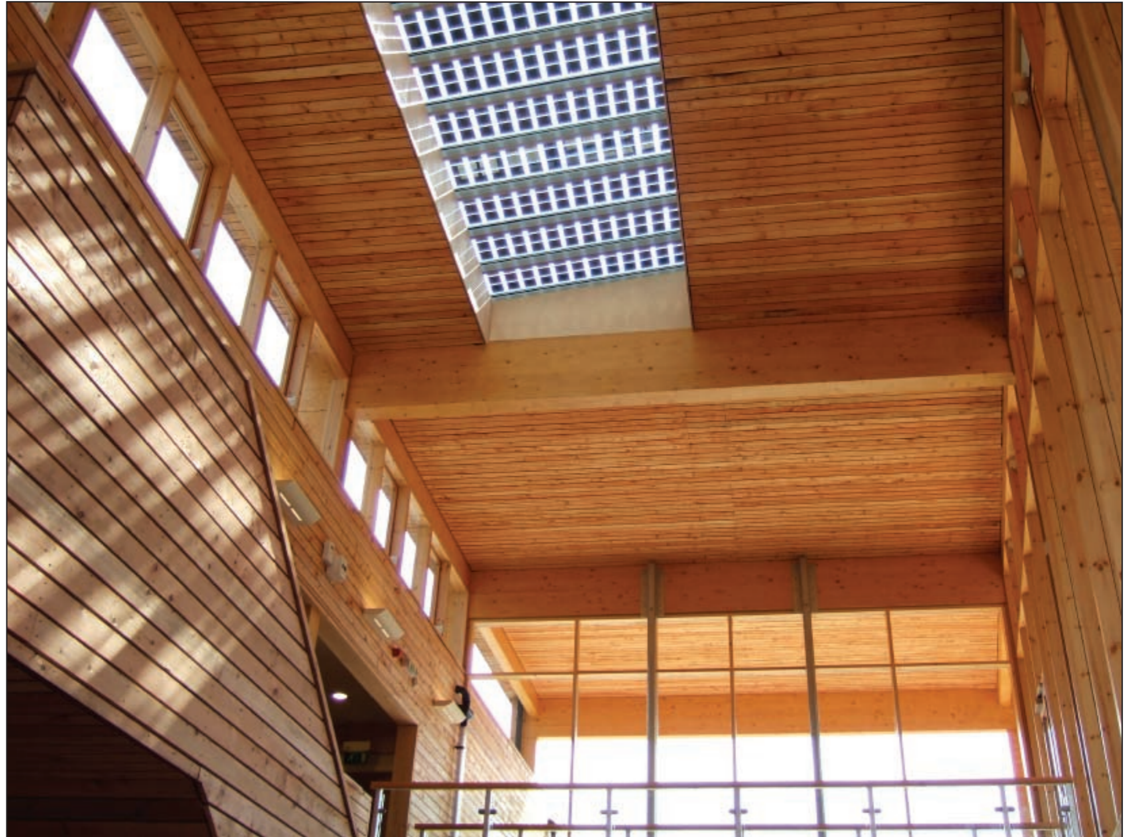
Thin-film photo voltaic array on roof light
