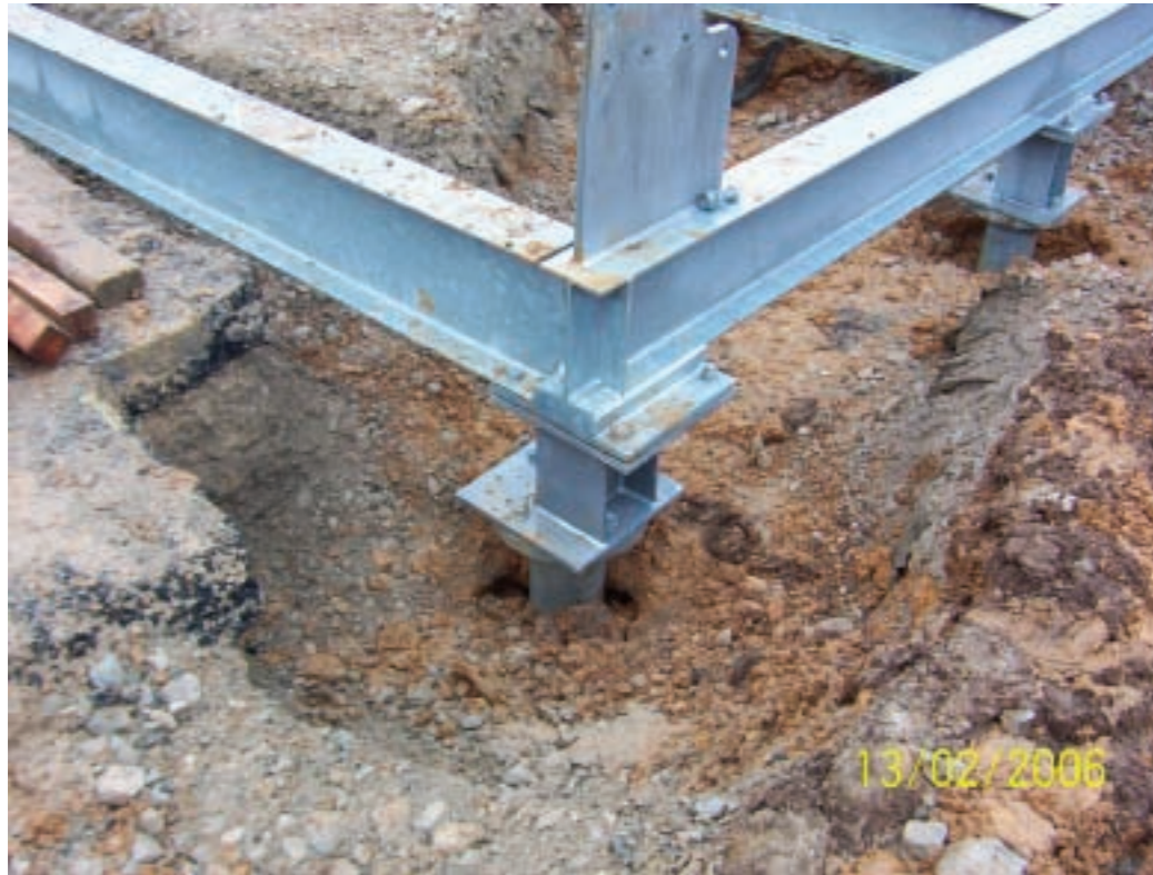
Screw piles and steel frame
