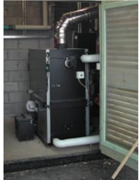
Above: Woodfuel boiler Below: Charterhouse Centre, Somerset PHOTOS: SW WOODFUELS
