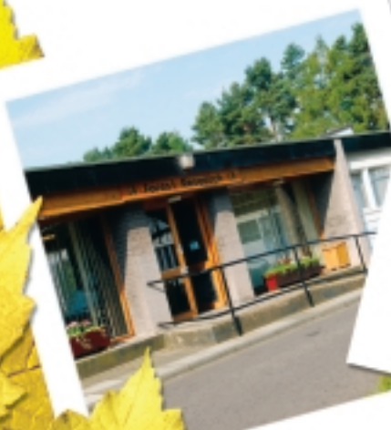
Entrance to the Northern Research Station at Roslin
