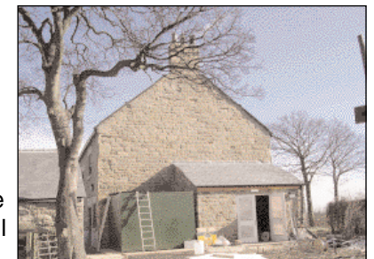
The boiler house and storage hopper at RSPB Oldmoor
