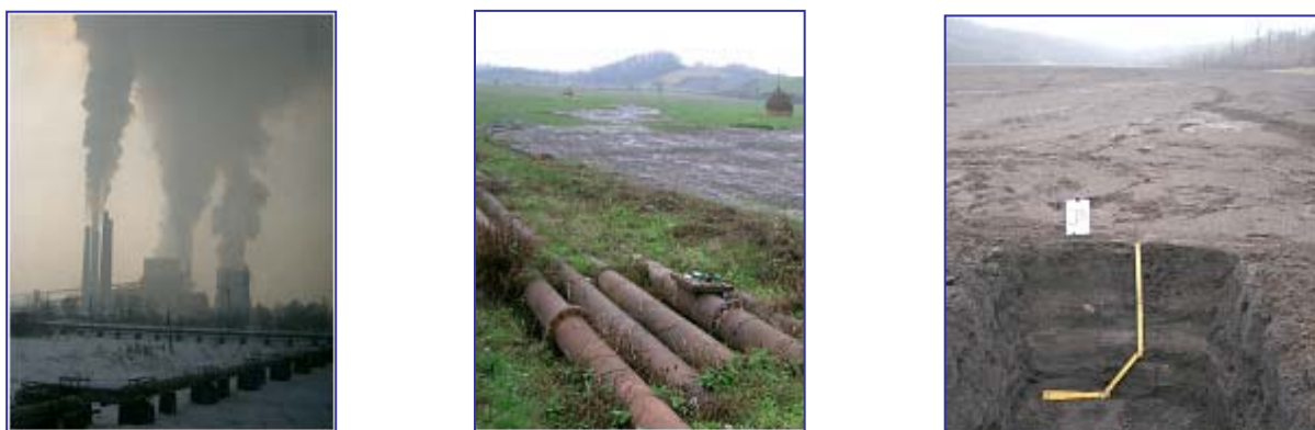
Figure 1. The thermo-electric power plant in Tuzla, pipelines for wet deposition of coal ash and an ash profile on a recently abandoned coal ash deposit.
