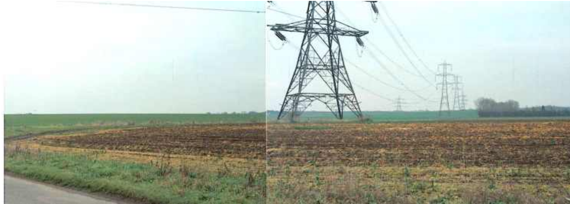
2. View from Church Road east
