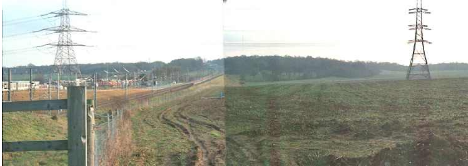
5. View from Henhurst Road near the CTRL works to Ashenbank Wood
